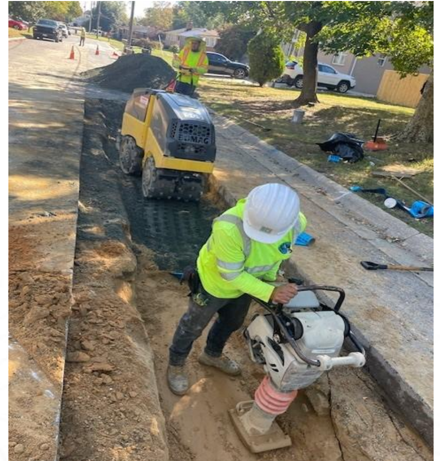
October 2025 - Crew is backfilling and compacting the trench following the water main installation
